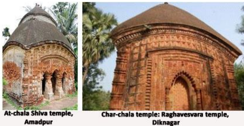
Figure 5. Showing Siva temple at Amadpur viii and Raghavesvara temple at Diknagar ix
