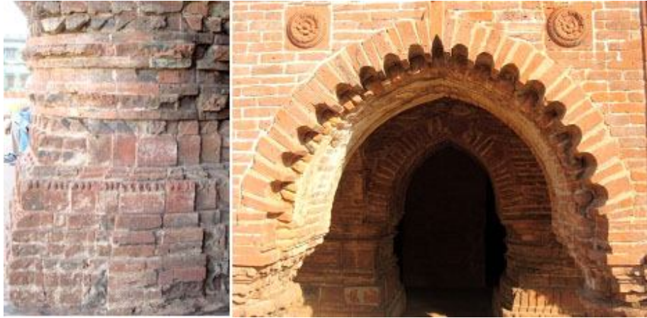
Figure11. Different sizes of brick were used according to the requirement.
