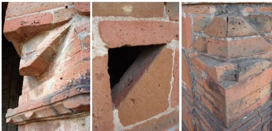
Figure13. Different sizes and shapes of bricks used to get the desired effect
