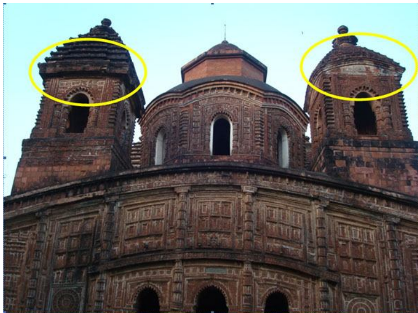
Figure 16. While conserving the Shyamrai temple one of the roof of the tower was made straight instead curvilinear form
