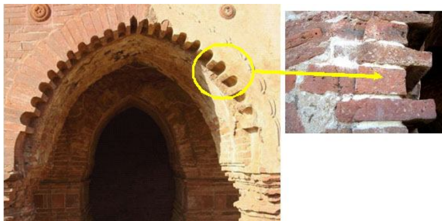
Figure12. In case of arch bricks are cut to form tapering voussoirs
