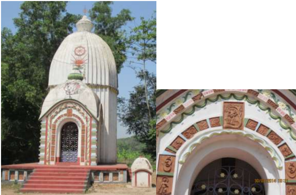
Figure 13 & 14: Brindavana Jiu Temple, Damodarapur (Front View), (Close-up of terracotta works)
