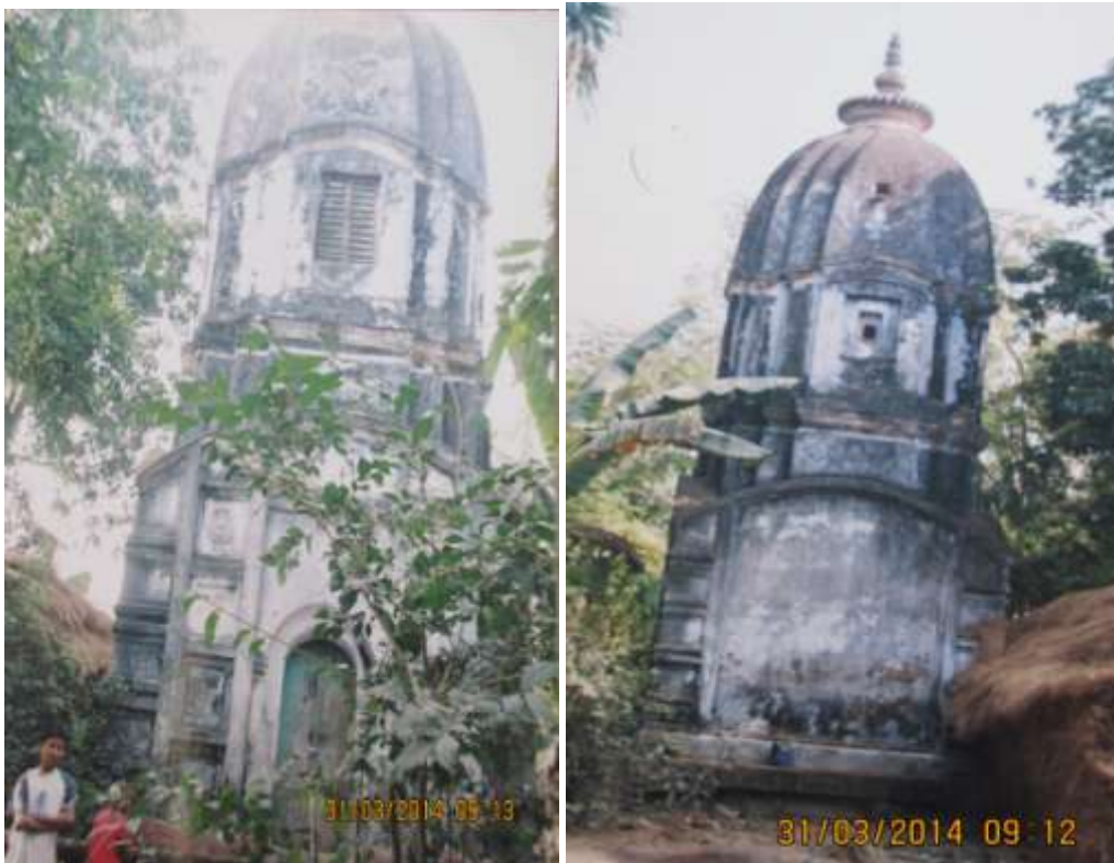
Figure 10: Siddheswara Siva Temple, Haripur (front view) Figure 11: (back view)
