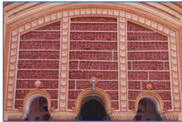
Main East Facade
